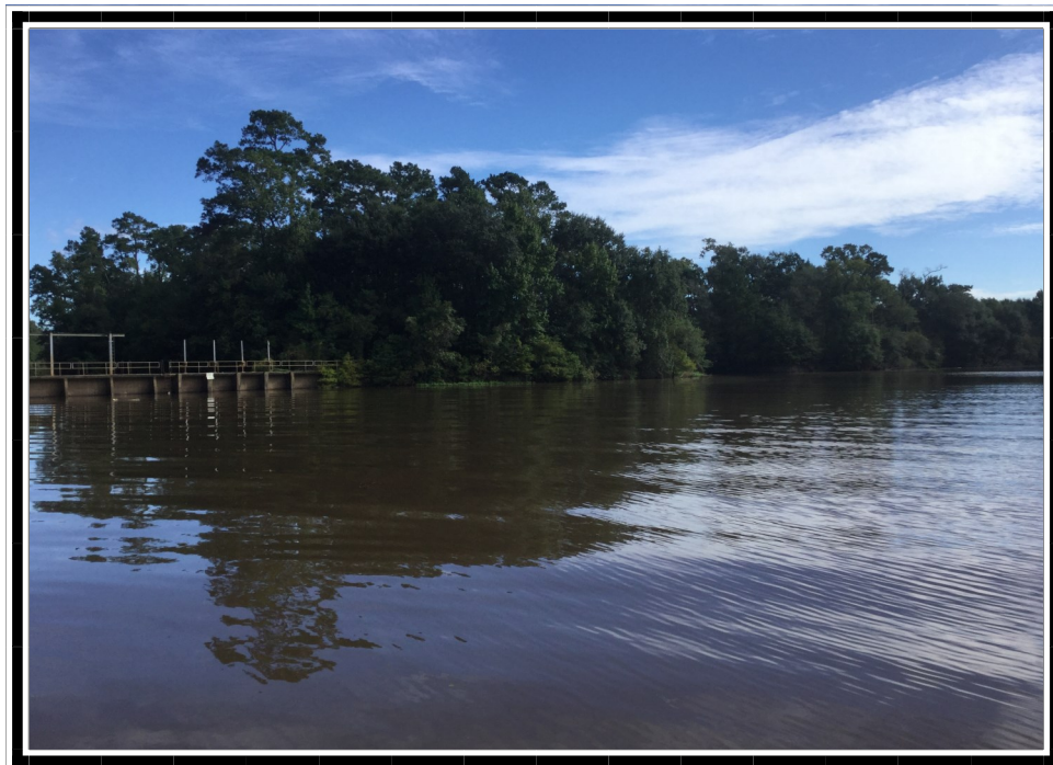
PINE ISLAND BAYOU AT LNVA LOWER PUMP STATION, 6.62 KM UP-STREAM OF NECHES RIVER CONFLUENCE 2.86 KM EAST OF US 69
