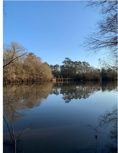
Figure 3.62 Station #10599: PIB @ LNVA 1st Pumping Station
