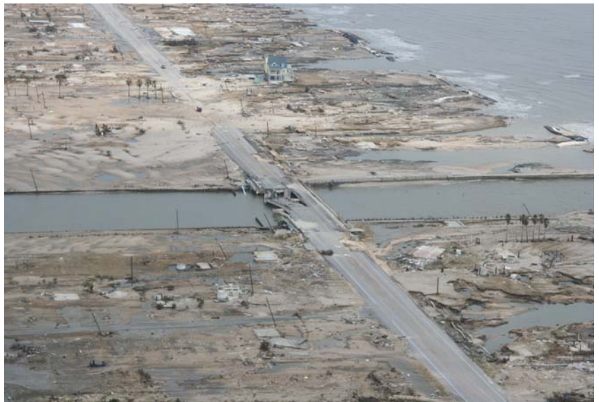
The Rollover Pass bridge on Hwy. 87 was severely damaged by Hurricane Ike’s storm surge estimated at 12 to 16 feet on the Bolivar Peninsula in Southeast Texas.
