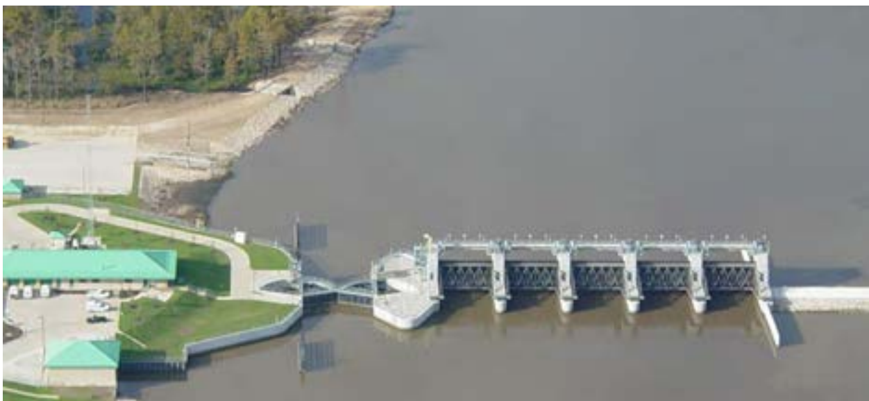
The Neches River Saltwater Barrier includes a laboratory, public boat ramps and public restrooms.
