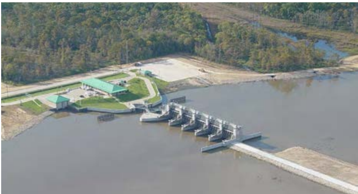
Aerial view of the Neches River Saltwater Barrier located in Beaumont, Texas
