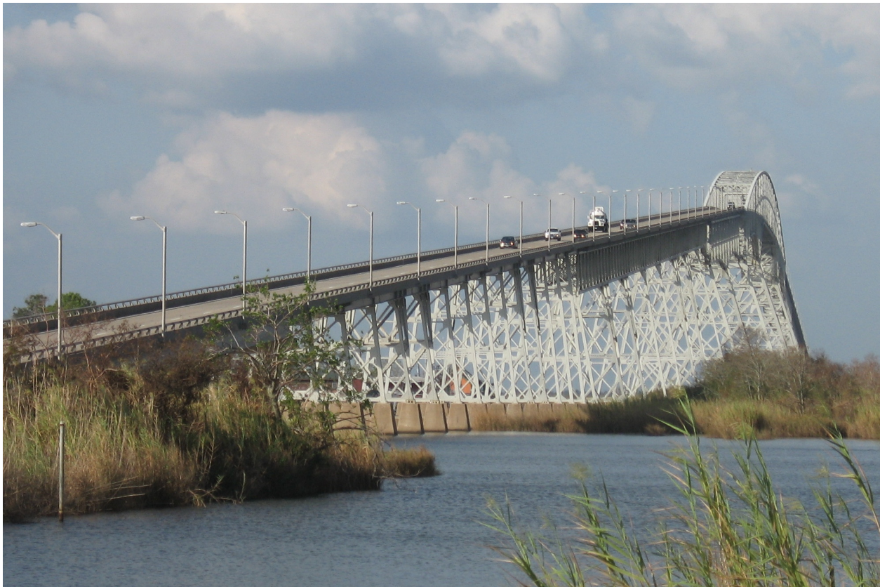
The Port Arthur-Orange Bridge (commonly known as Rainbow Bridge) is a massive cantilever and continuous steel truss over the Neches River. – Texas Historical Commission at http://www.thc.state.tx.us
