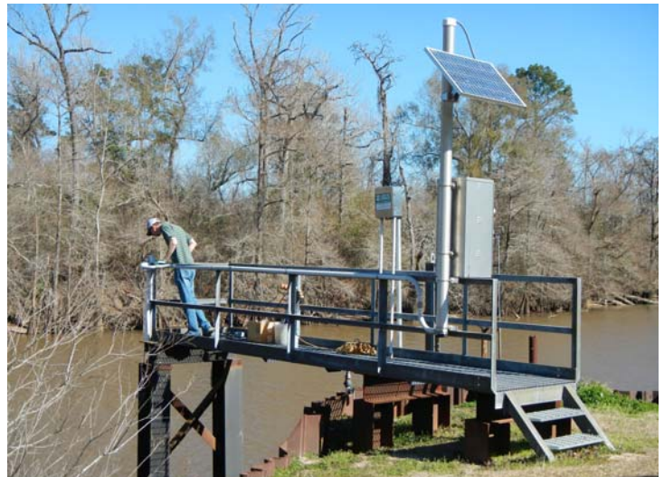
Real-Time Monitoring Station on Pine Island Bayou (CAMS 749)
