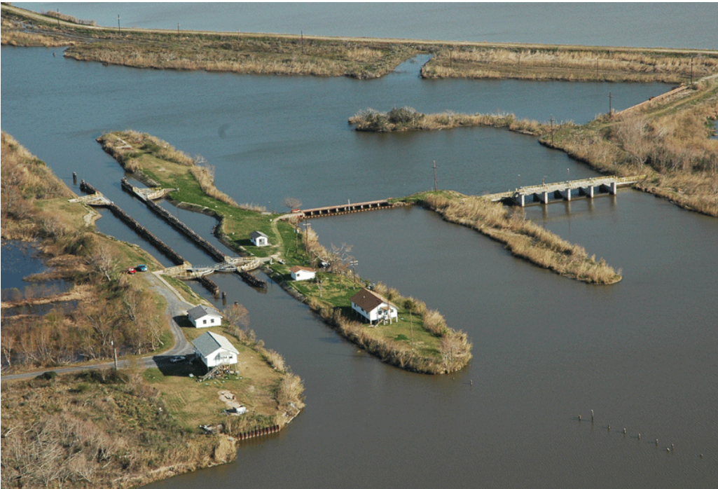
Saltwater barriers and navigational locks at the Sabine-Neches Navigation District's Taylor Bayou facility control saltwater intrusion in Taylor and Hillebrandt Bayous from the Intracoastal Waterway. (photo provided by SNND)
