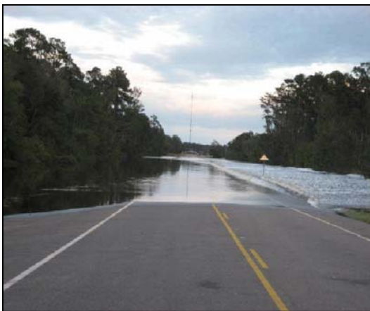
Figure 1. Village Creek flows over Hwy. 327 near Silsbee, TX on Oct. 21, 2006.
